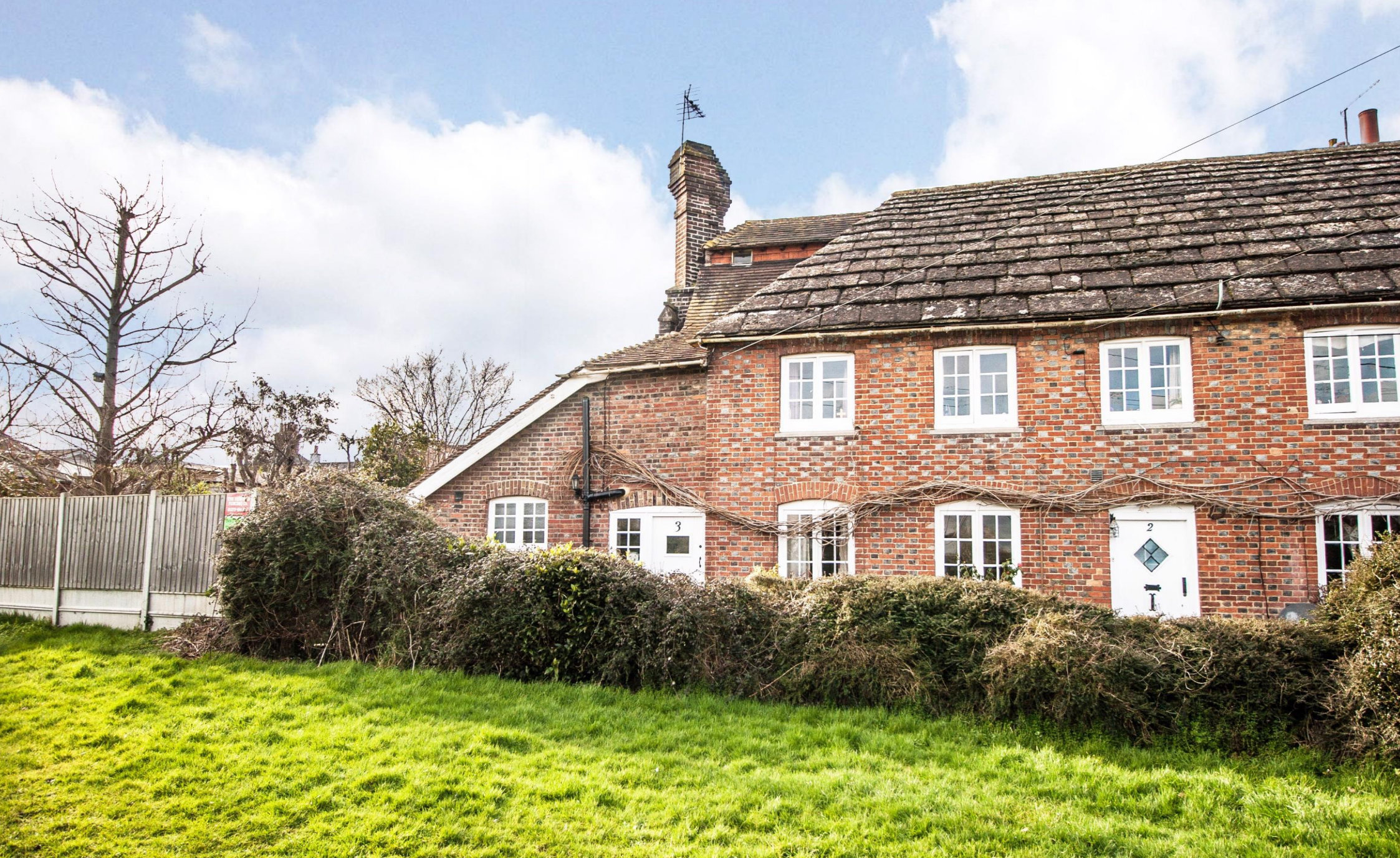
3 Cedar View, Nep Town Road, Henfield, West Sussex.
